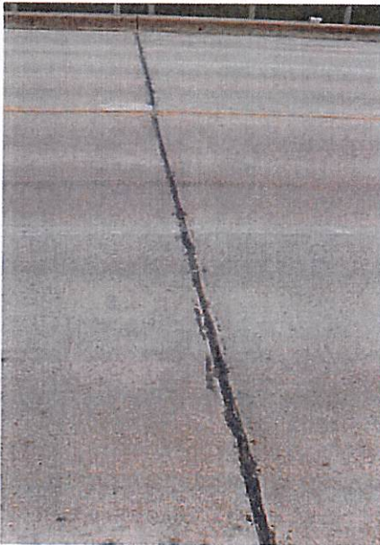
Figure 18: Expansion Material Deteriorating
