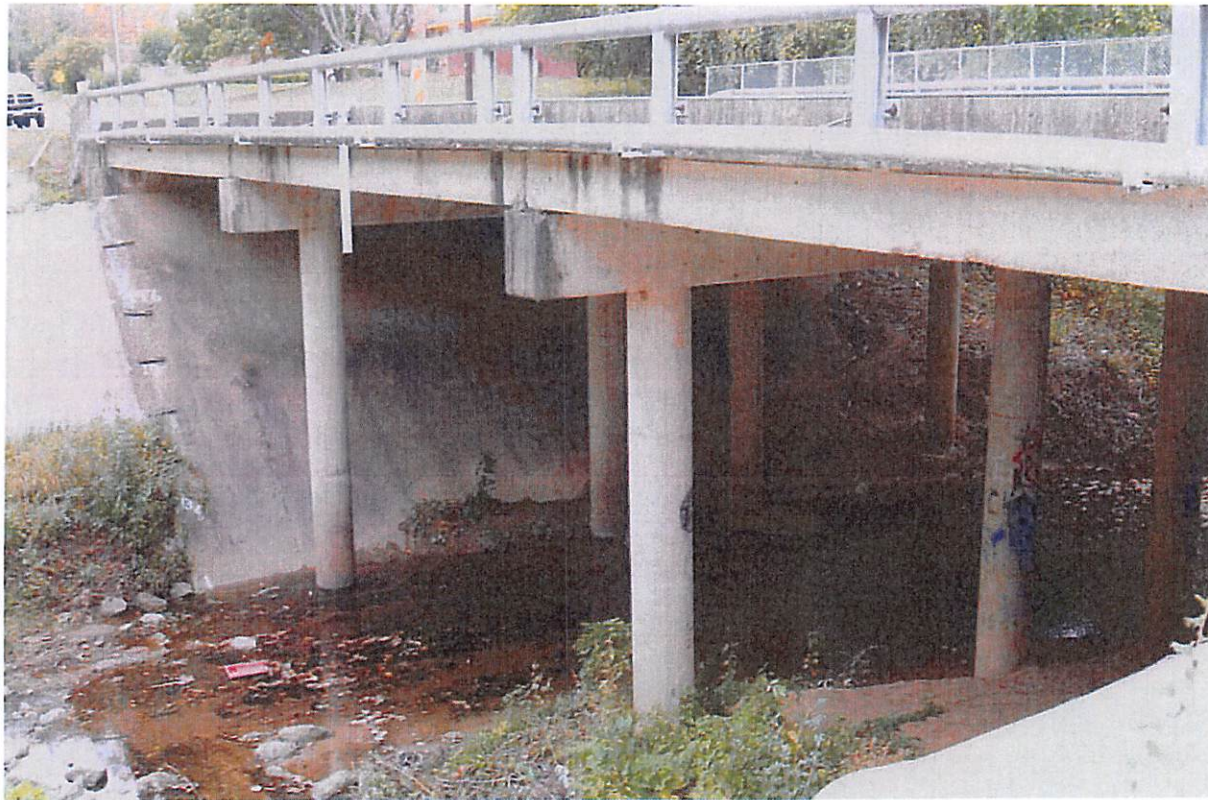
Figure 26: Concrete Columns and Bents in Satisfactory Condition
