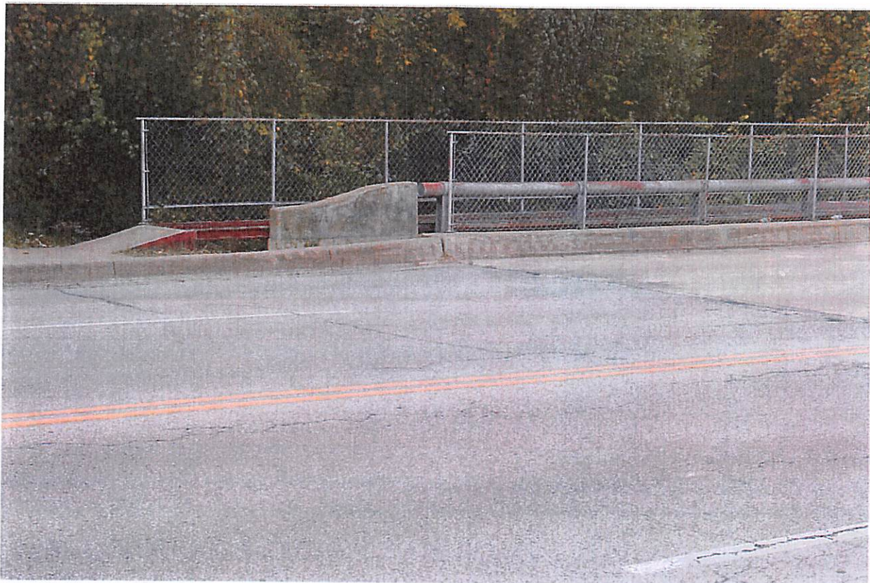
Figure 23: Pedestrian Walkway is Not ADA Compliant
