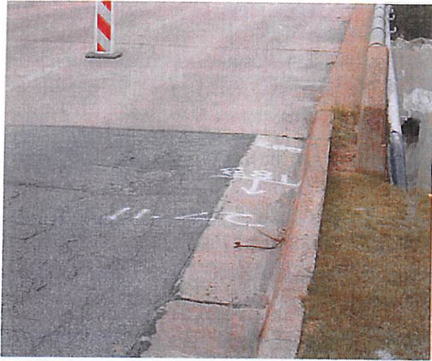
Figure 21: No MBGF and Failing Pavement at Northbound Lanes
