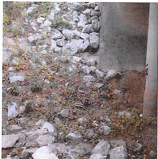
Figure 29: Buried RCP Pipe and Loose Rock Riprap
