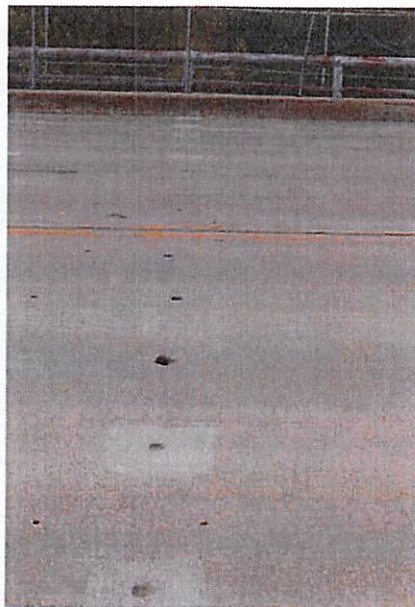
Figure 19: Form Holes are Inadequately Maintained
