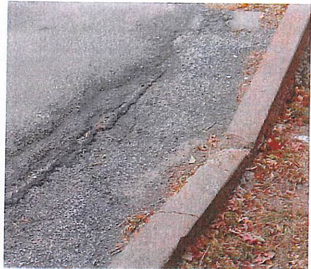
Figure 22: Broken Approach Slab at Southbound Lanes
