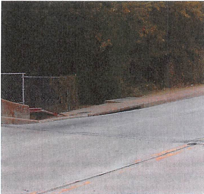
Figure 24: Failed Approach Slab and Curb Inlet due to Loss of Support
