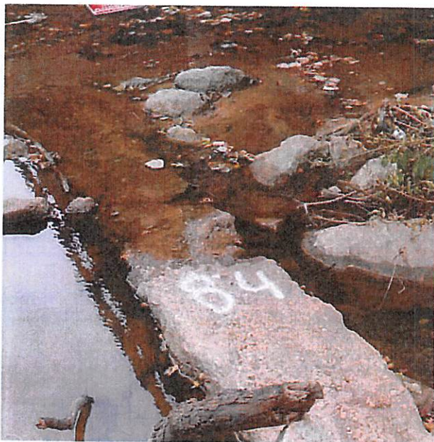
Figure 28: Exposed Concrete Encasement
