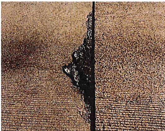
Photo 1: Damaged armor joint, northbound lanes, north abutment
