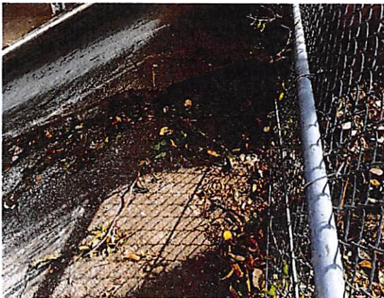
Photo 6: Severe undermining of abutment riprap, southbound lanes, south abutment
