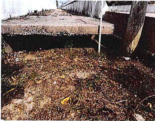
Photo 5: Severe undermining of approach slab and sidewalk, southbound lanes, south abutment
