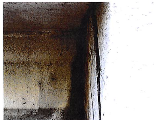
Photo 4: Damaged abutment backwall (spalling), southbound lanes, south abutment
