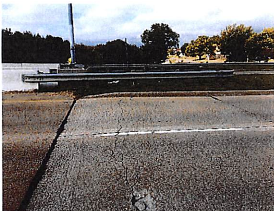
Photo 2: Damaged approach slab, northbound lanes, north abutment
