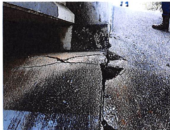
Photo 3: Compromised abutment riprap, southbound lanes, south abutment
