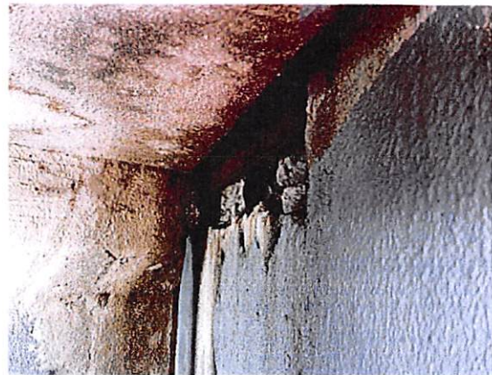
Photo 7: Honeycombing at armor joint on abutment backwall, southbound lanes, south abutment
