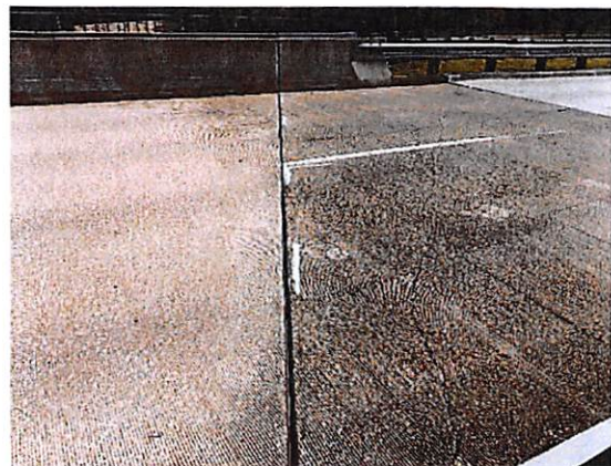
Photo 8: Approach slab cracking, southbound lanes, south abutment
