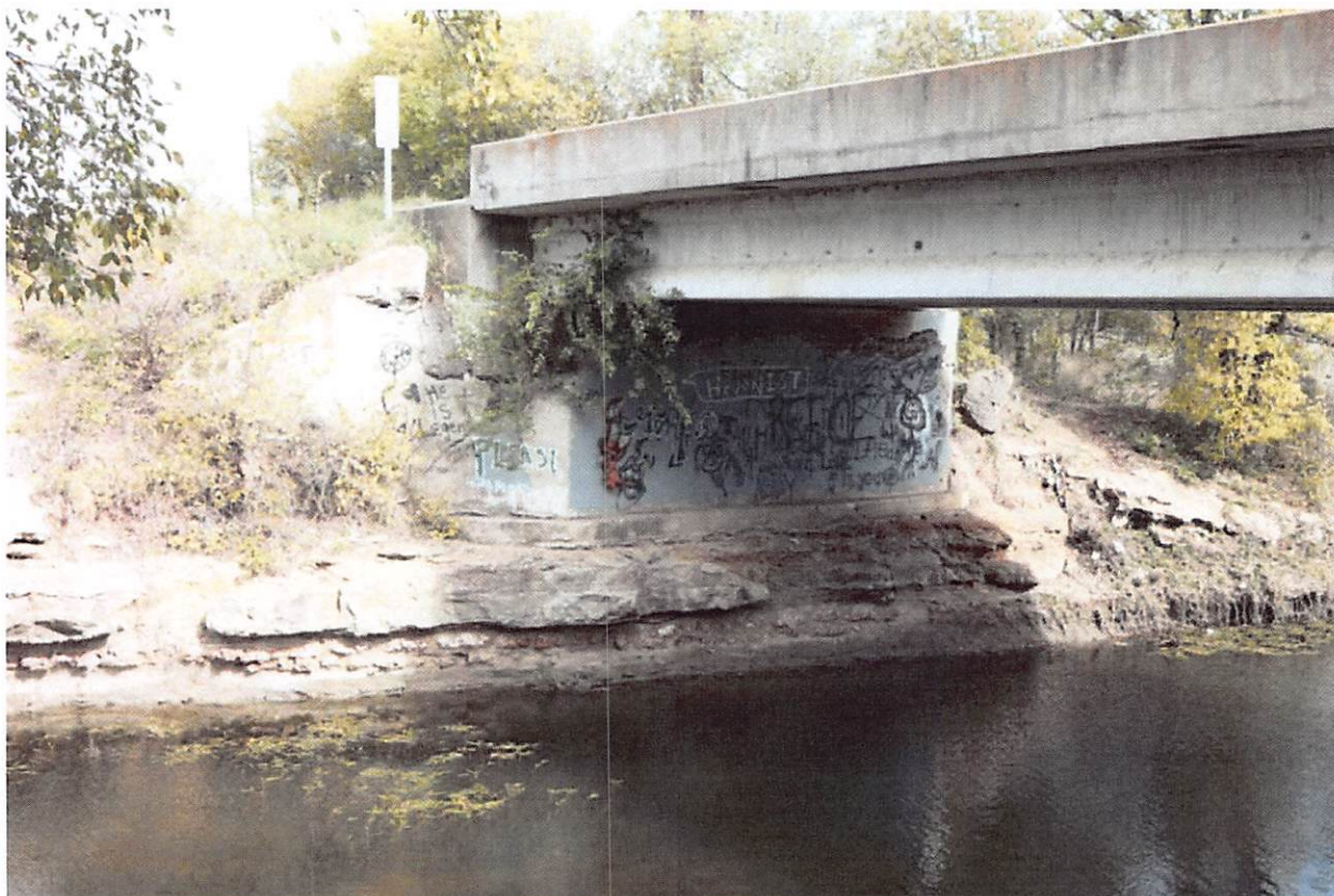
Figure 51: Channel Sides Supporting Original Abutments are Eroding
