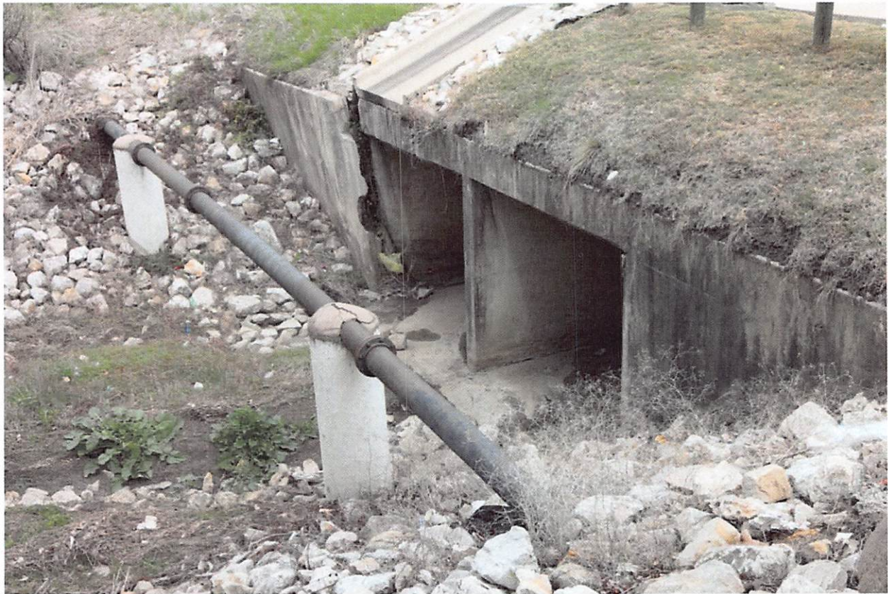
Figure 31: Western Headwall Showing Failed Wingwall
