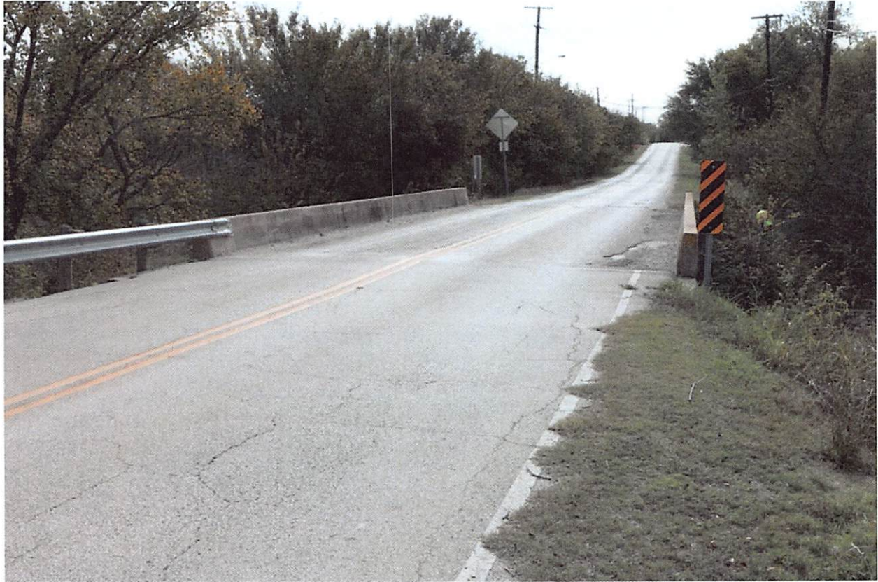
Figure 46: Only One Section of MBGF - Looking South
