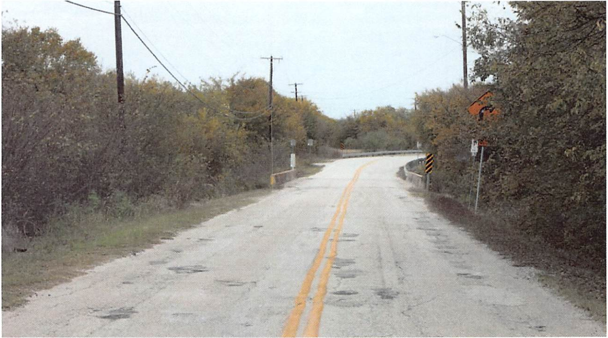
Figure 47: Road Surface with Many Potholes - Looking North
