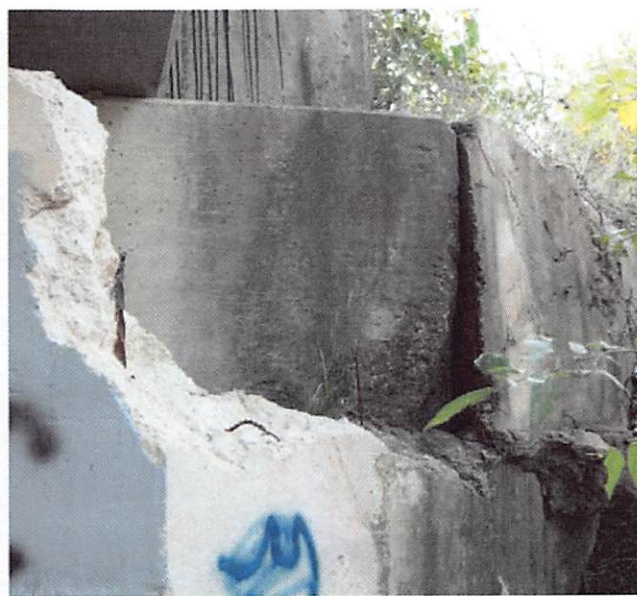
Figure 53: Pier Cap for Current Bridge is Integral with Original Bridge Abutment
