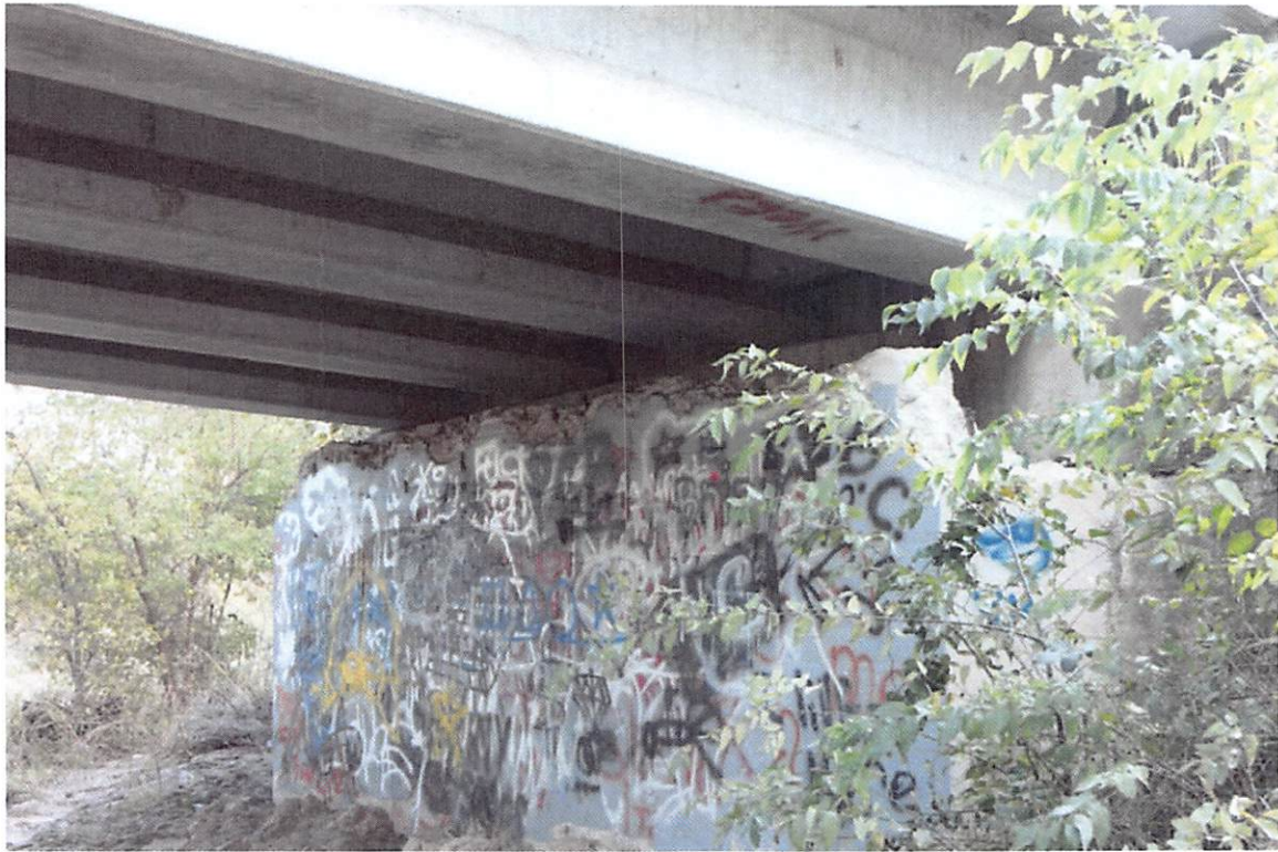
Figure 49: Original Abutment from Earlier Bridge is Still Present (South Side)
