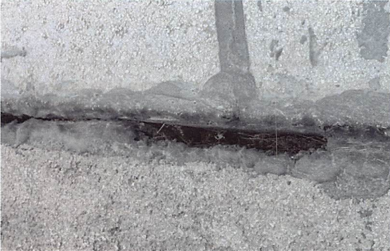
Figure 42: Separation at Inlet
