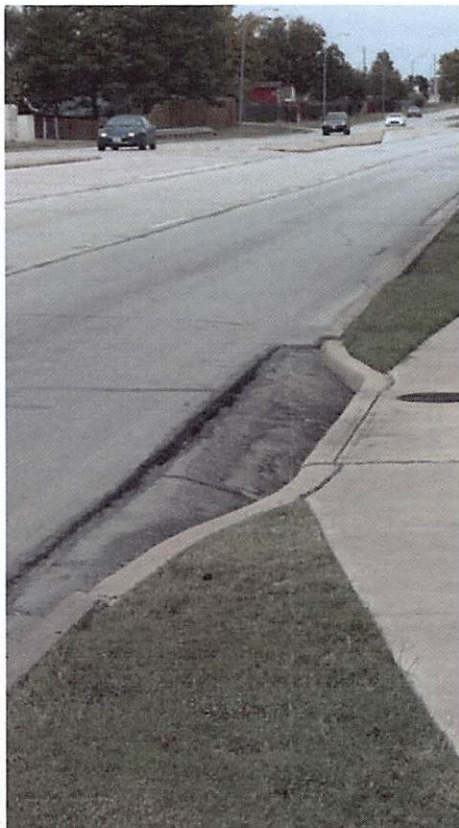
Figure 36: Curb Inlet has Moved
