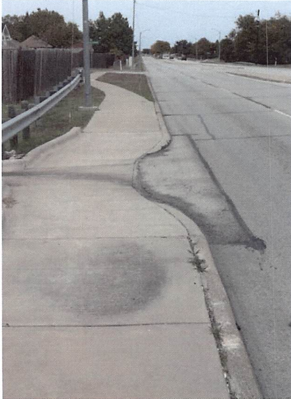
Figure 32: Drainage Flume (Looking North)
