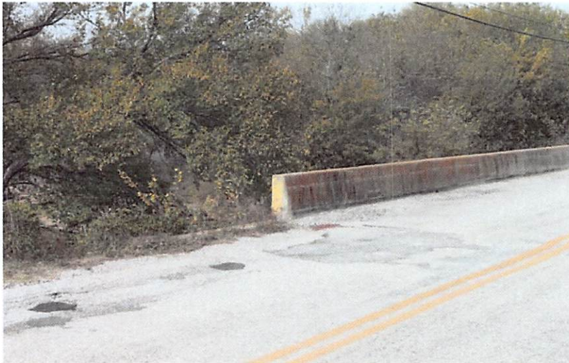
Figure 48: Failed Pavement has been Patched Multiple Times
