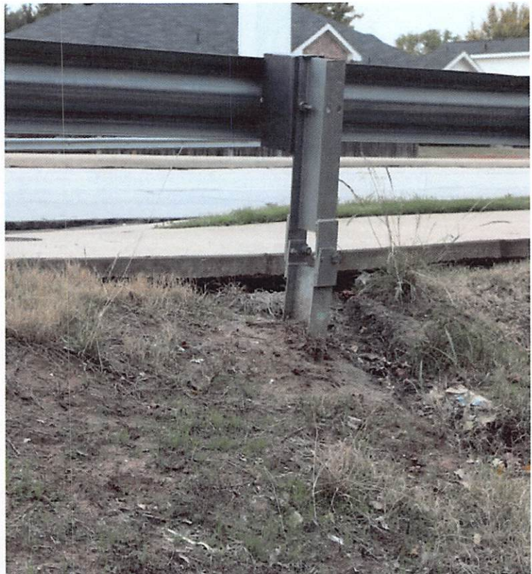
Figure 37: Erosion Behind Inlet Under Sidewalk
