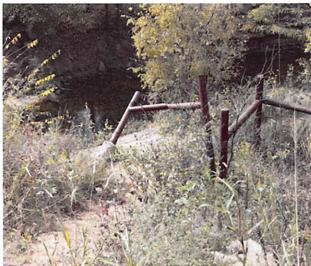
Figure 55: Erosion Down Banks has Caused Fence Posts to Wash Out
