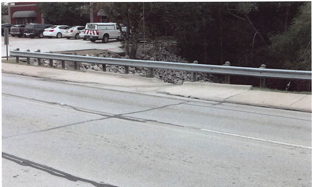
Figure 34: Drainage Flume, MBGF, and Channel Riprap (Looking West)
