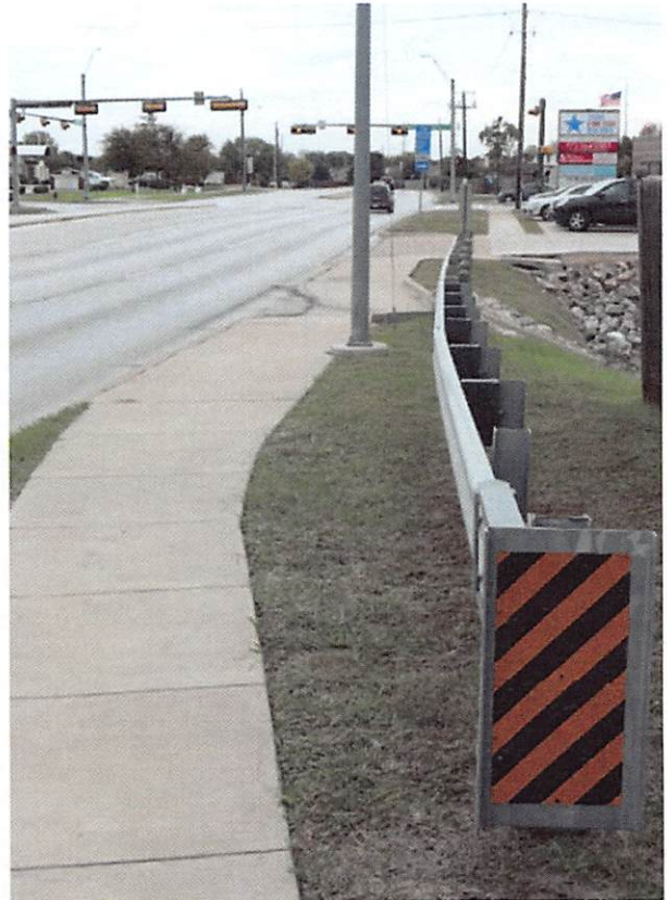
Figure 33: SGT for Southbound Traffic
