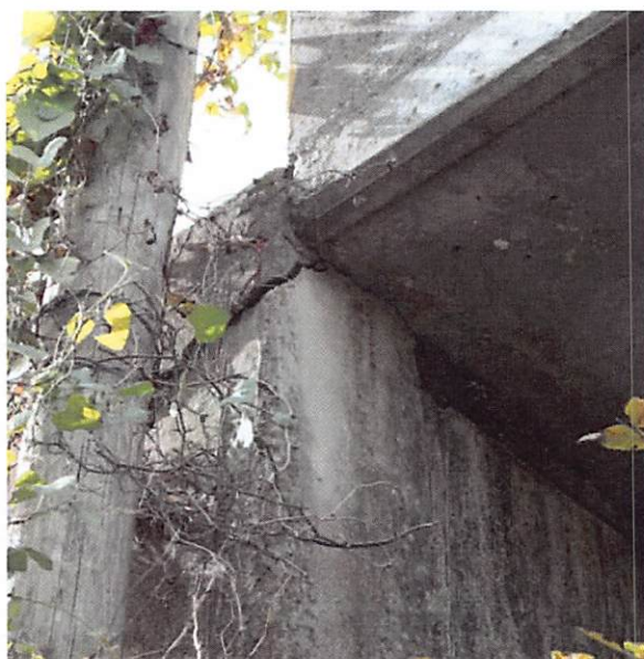
Figure 52: Concrete Abutment Backwall is Cracked
