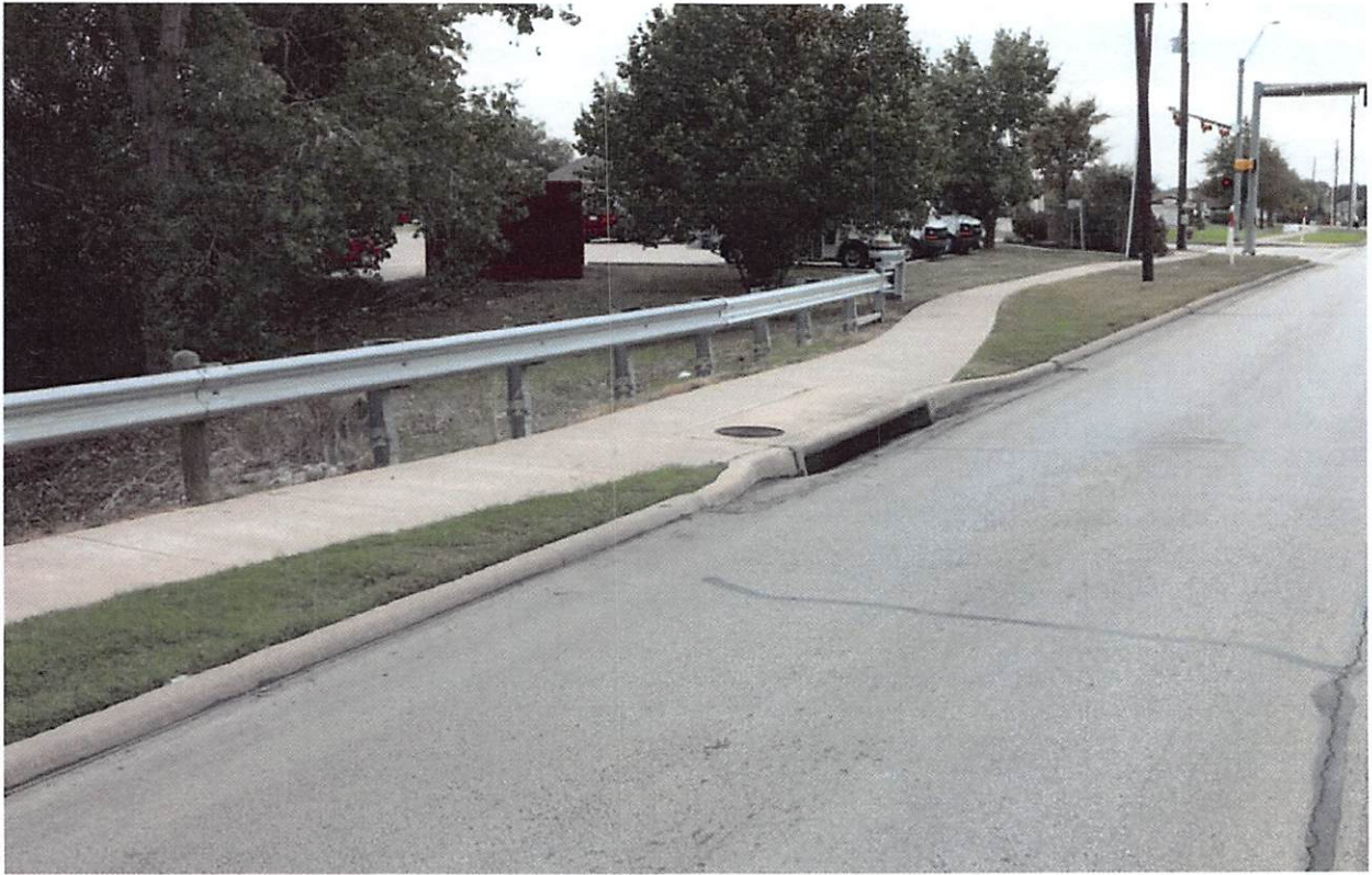
Figure 35: Curb Inlet on East Side (Looking South)
