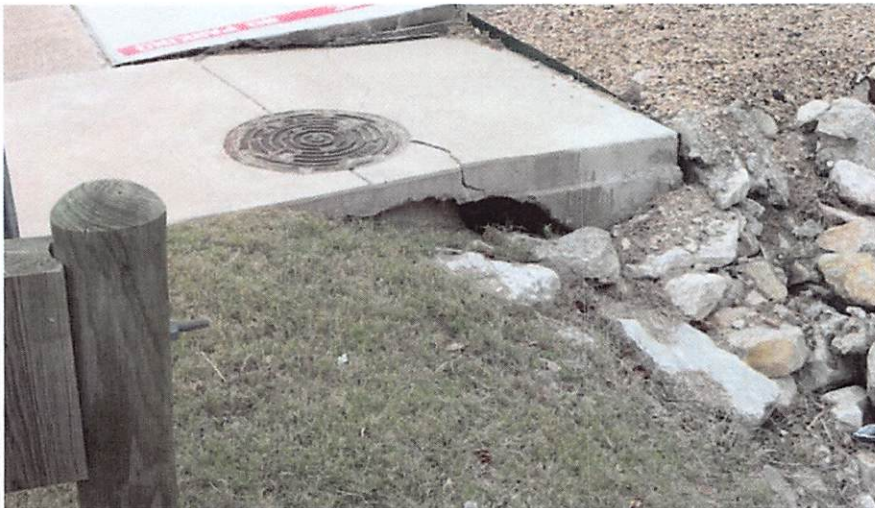
Figure 44: Erosion under Sidewalk Near Adjacent Parking Lot
