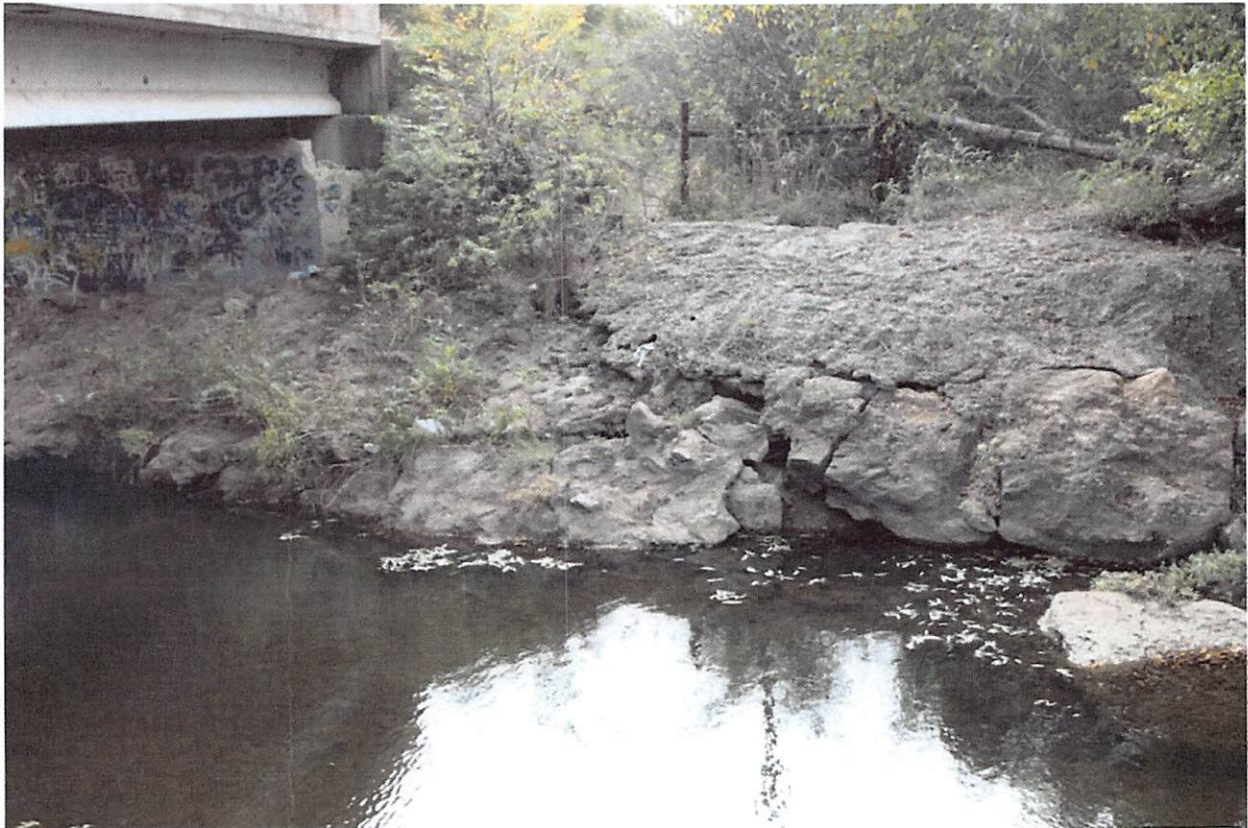
Figure 54: Grouted Riprap is Undermined and Losing Support
