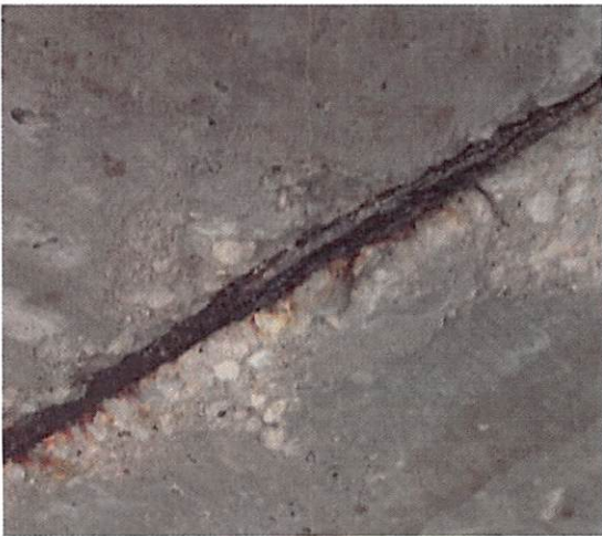
Figure 43: Exposed and Corroded Reinforcement
