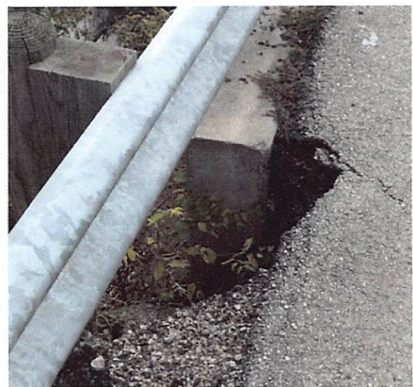
Figure 56: Erosion Near Approach Slab Undermining HMA Pavement
