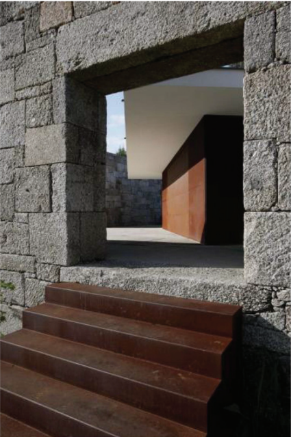
EXAMPLES OF STONE MASONRY FACADE
